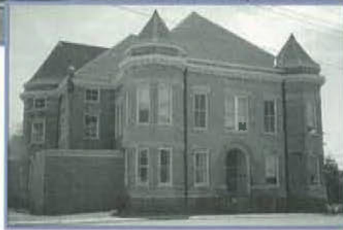
Rear view of 1899 Conecuh County Courthouse
