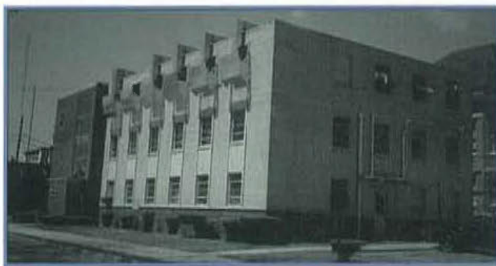
Front and side view of 1958 addition to Conecuh County Courthouse
