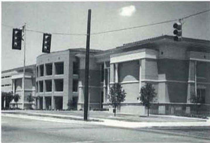
Front view of new Etowah County Judicial Complex
