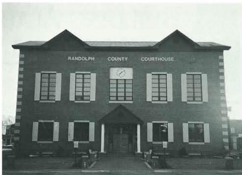
Randolph County Courthouse, after completed restoration
