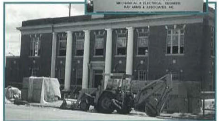
Eufaula Courthouse during renovations
