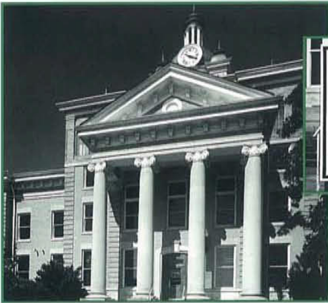
Close-up view of courthouse facade
