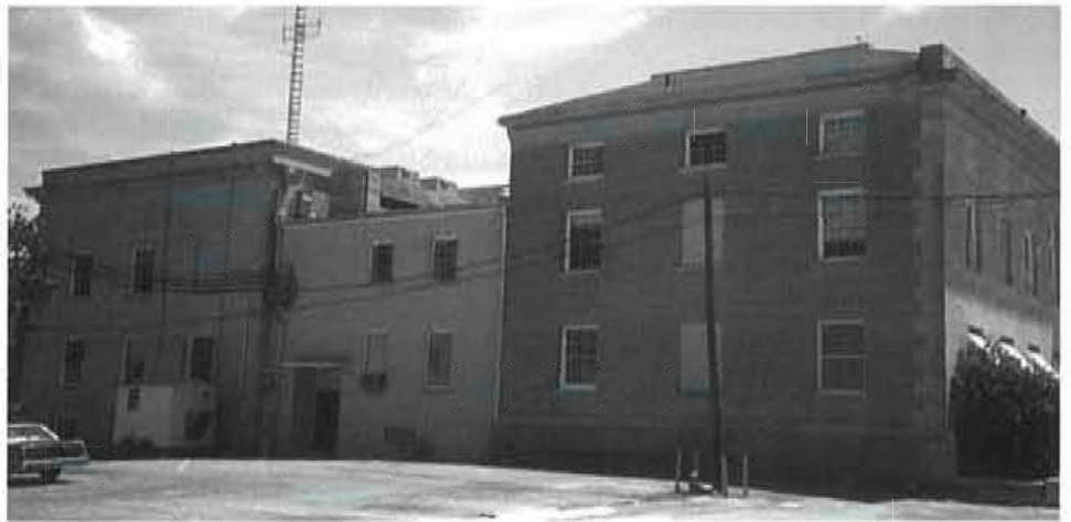
Rear of courthouse showing additions over the years
