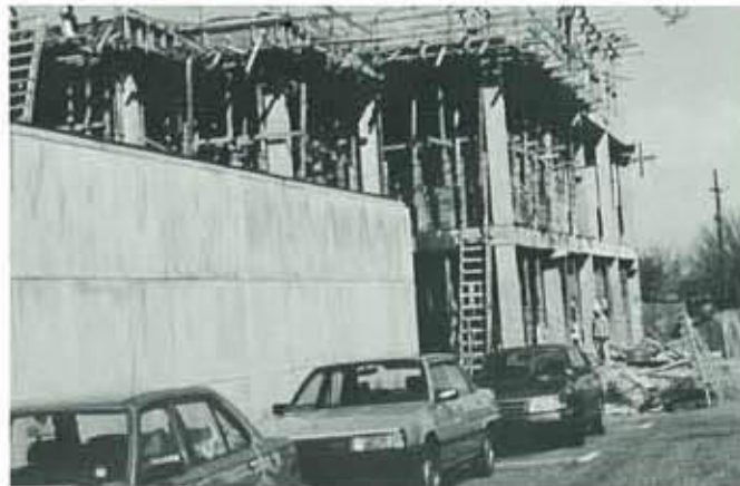
February: Forming columns for second to third floor.
