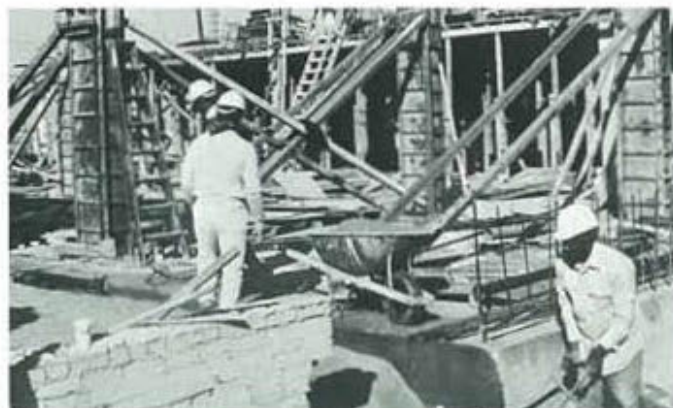
January: Pouring slab and forming columns for first to second floor.
