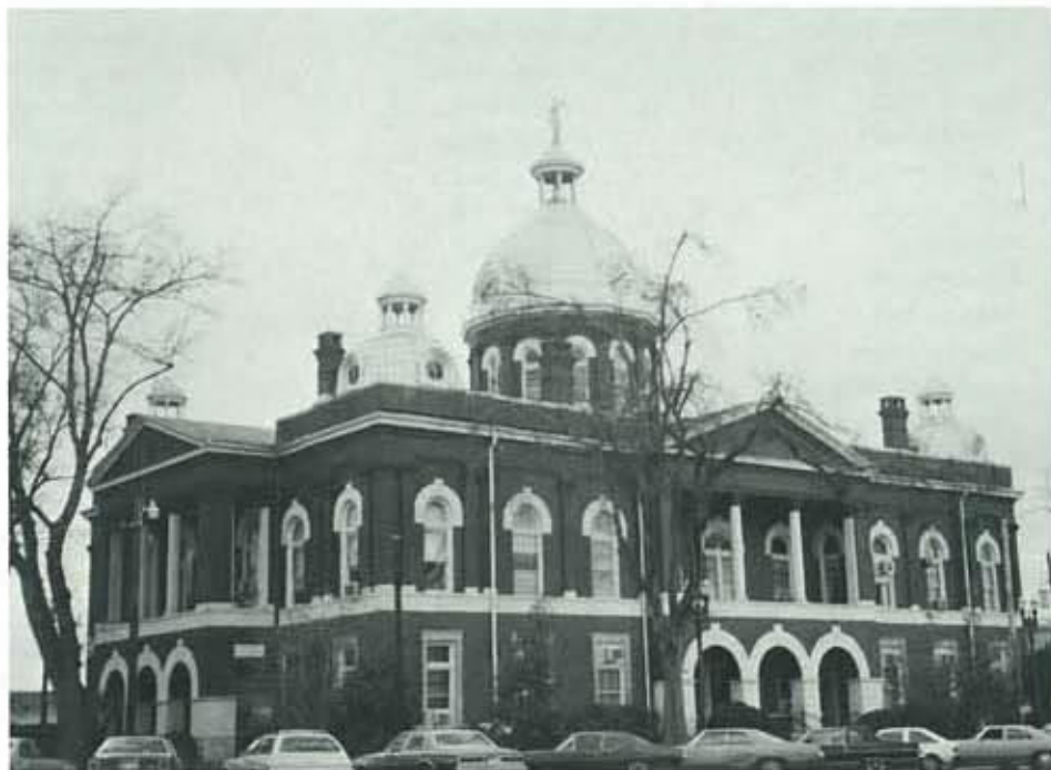
Chambers County Courthouse, following restoration
