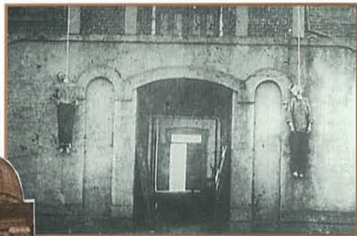
John Hipp and Charles Kelby Butler — County courthouse 1892
