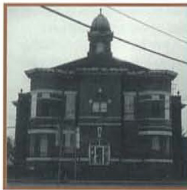
Rear of courthouse
