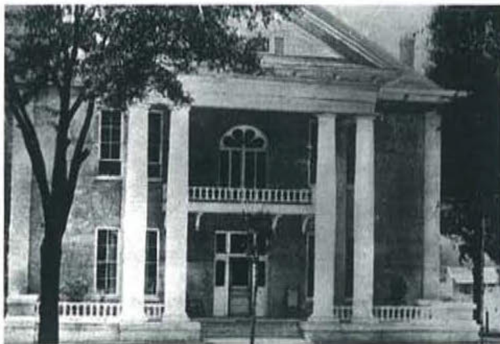
Courthouse after renovation into residence for C.H. Conoley
