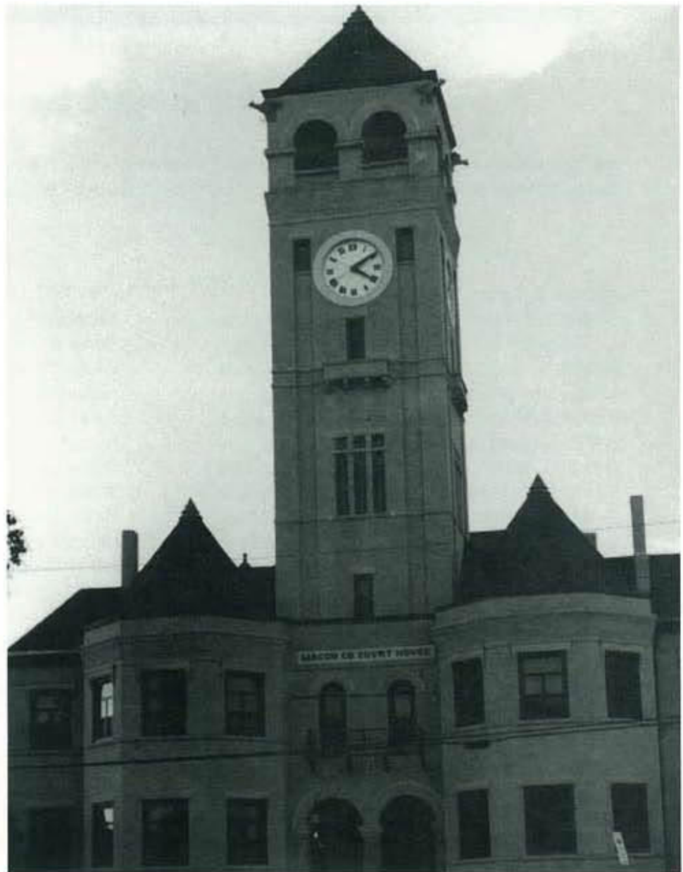
A view of the main or south facing entrance after renovation
