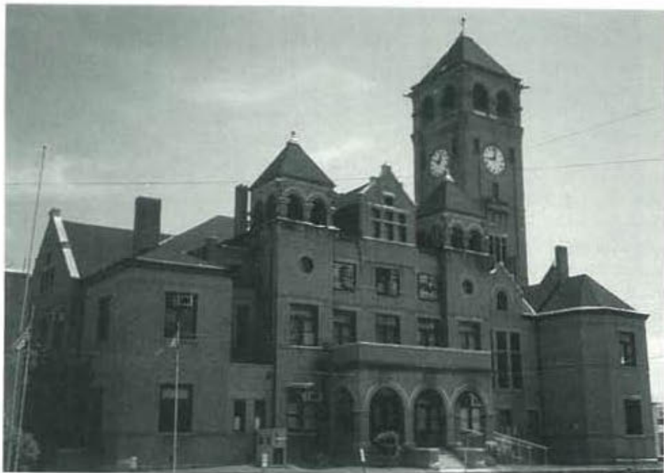
The west side of the Macon County Courthouse shows fire damage from 1885.
