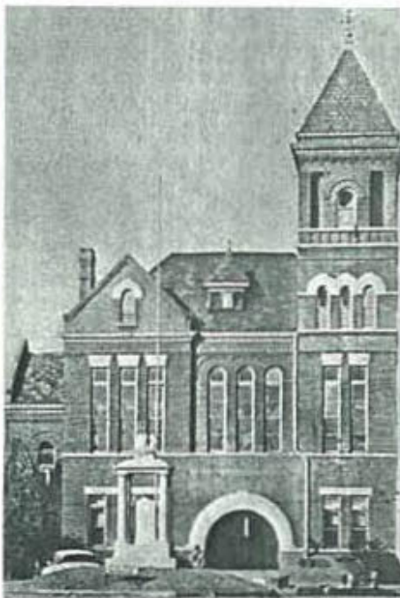
Photo of Clarke County Courthouse, 1899 to 1955
