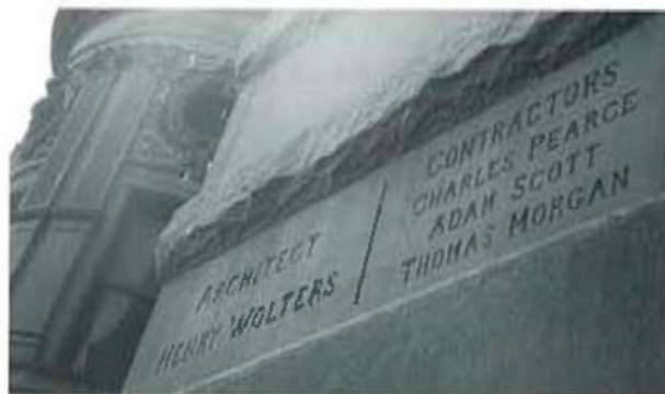
Cornerstone showing architects and contractors
