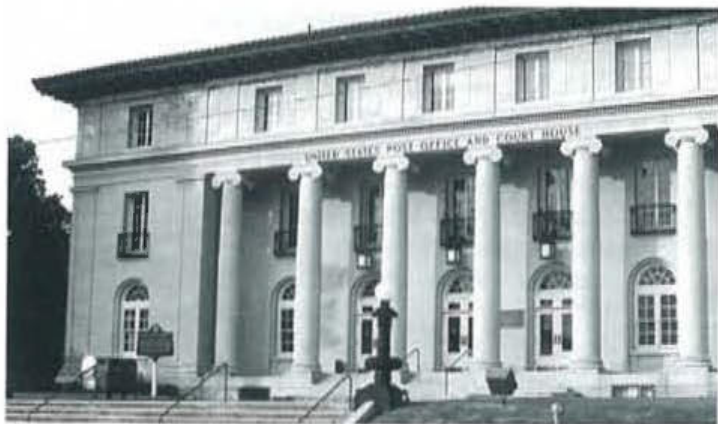
Justice John McKinley Federal Building, which serves as the U.S. Post Office and Courthouse, Florence, Alabama
