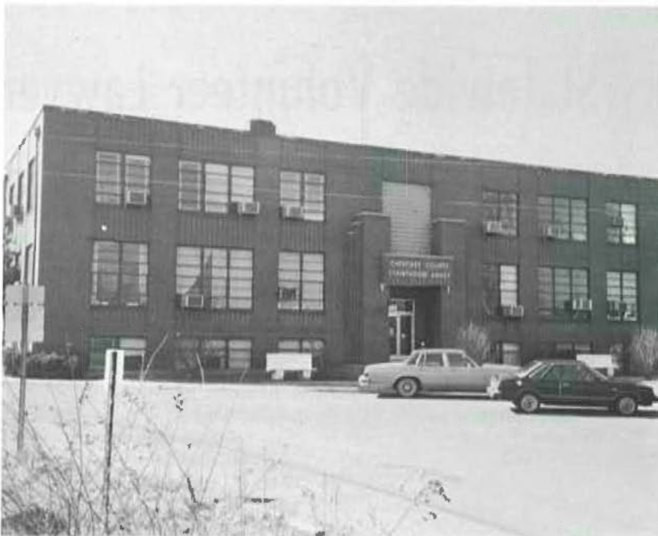
Cherokee County Courthouse Annex
