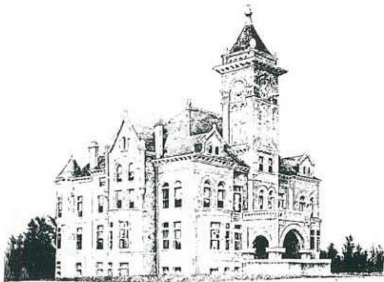
Courthouse number four, located in Linden, was destroyed by fire in 1965.
