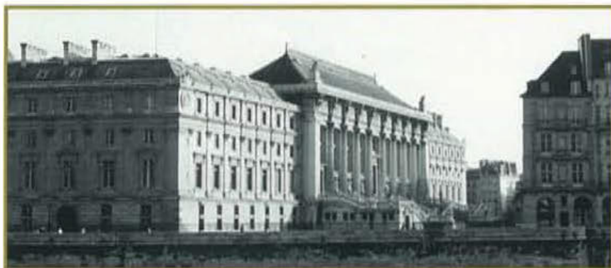
Main facade of Palais de Justice
