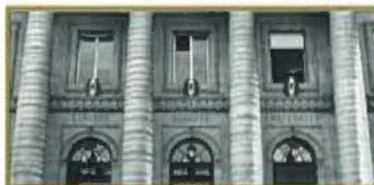
Working entrance to Palais de Justice
