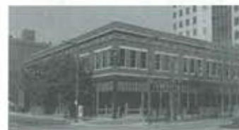
THE CLARK BUILDING
