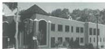
2146 HIGHLAND AVENUE BUILDING
